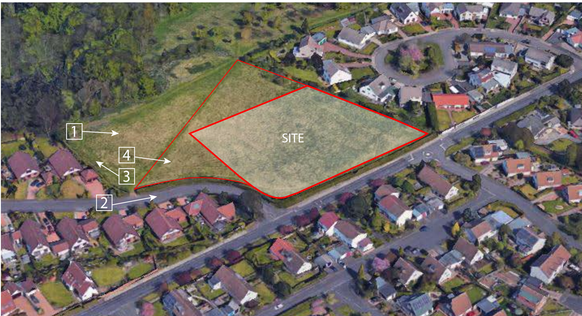
Aerial view of existing site
